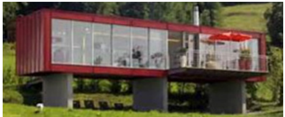
Cargo containers converted to living units.
