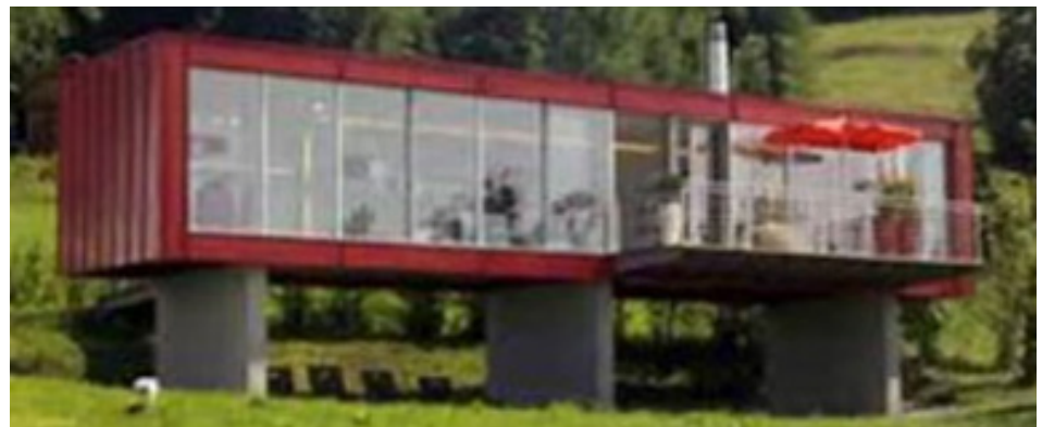
Cargo containers converted to living units.
