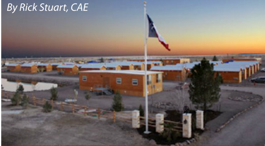
The Pecos Lodge, an impressive man camp facility owned and operated by Target Logistics, in Pecos, Texas.
