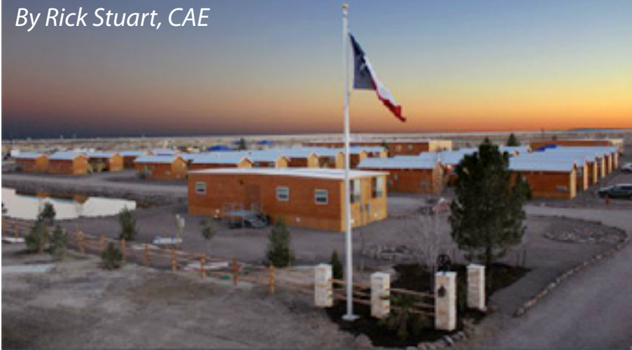
The Pecos Lodge, an impressive man camp facility owned and operated by Target Logistics, in Pecos, Texas.
