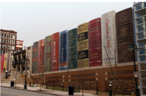
Kansas City, Mo., Central Library parking garage
